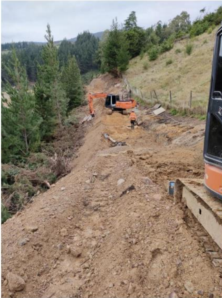
Figure 1 – Geotechnical stabilisation works being implemented above the airspace excavation works
