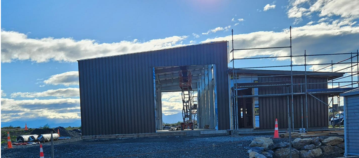
Figure 3: Facilities/Workshop Building Progress
