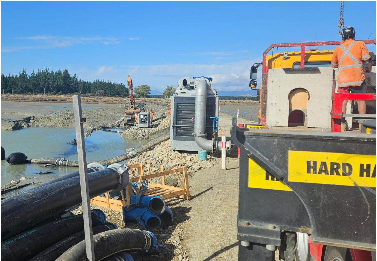
Figure 2: Pipework installation alongside Bell Island Causeway
