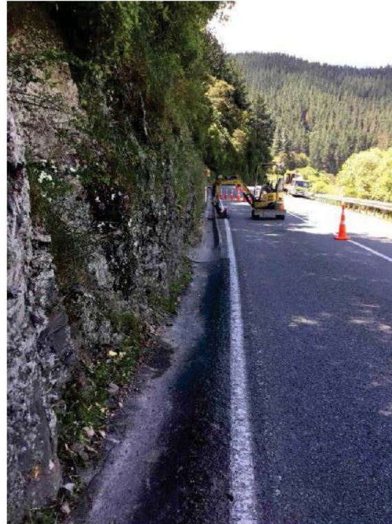
Lined channel cleaning on the Whangamoa's
