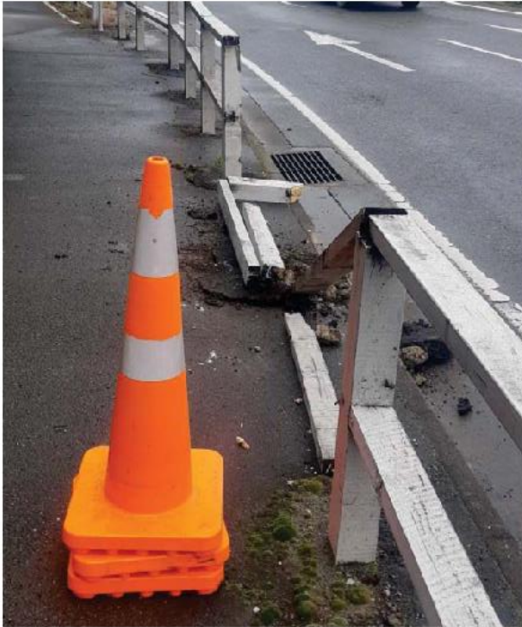
Slight rail damage at Quarantine Rd roundabout
