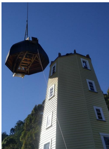
Windmill repairs on the dome, Founders Park, Nelson.
