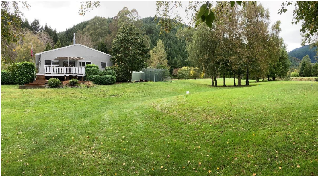
Figure 3: View southeast towards proposed hub site, showing Waahi Taakaro Golf Club House.
