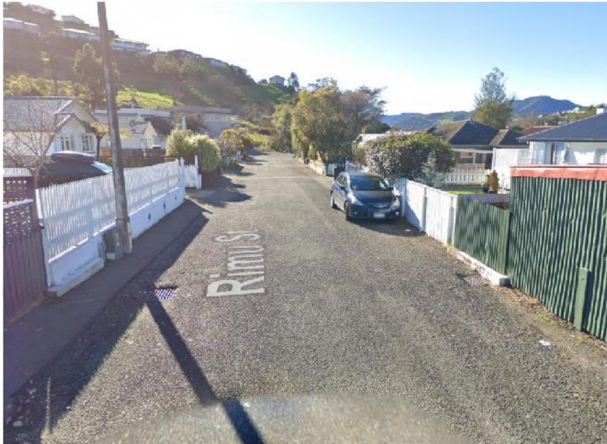
Figure 3: Rimu Street showing footpath on one side of the road with no delineating curb and channel
